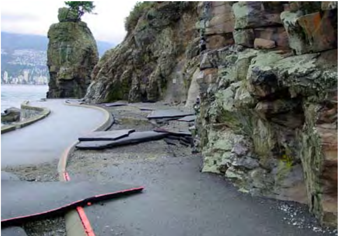
Seawall damage
