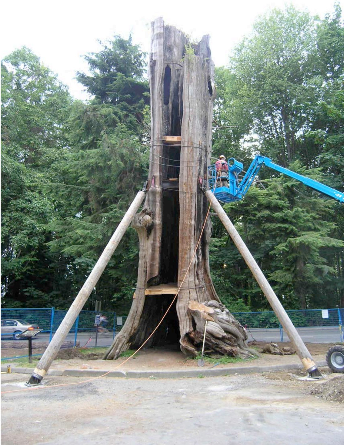
Figure 9. View of stabilized Hollow Tree from east showing two (2) struts and two (2) cables. (RC July 25, 2008)
