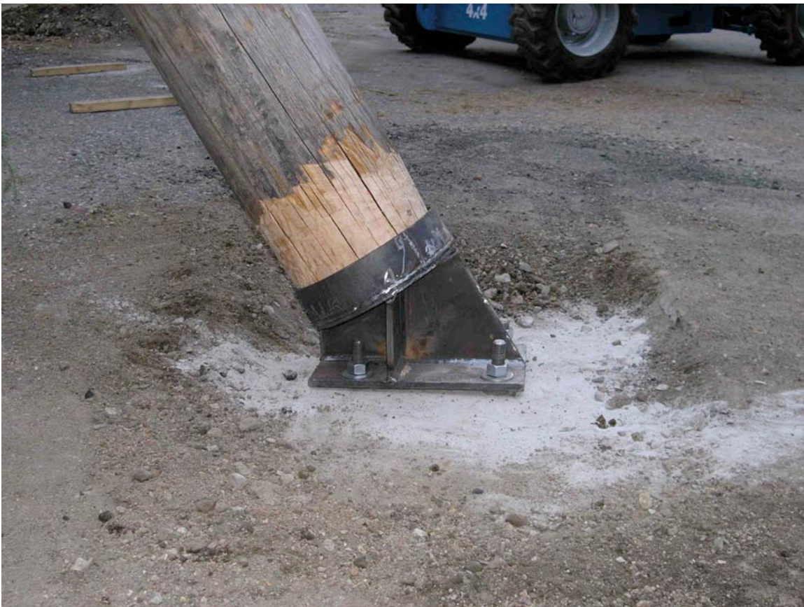
Figure 4. Base plate for south strut. (RAC July 25, 2008)
