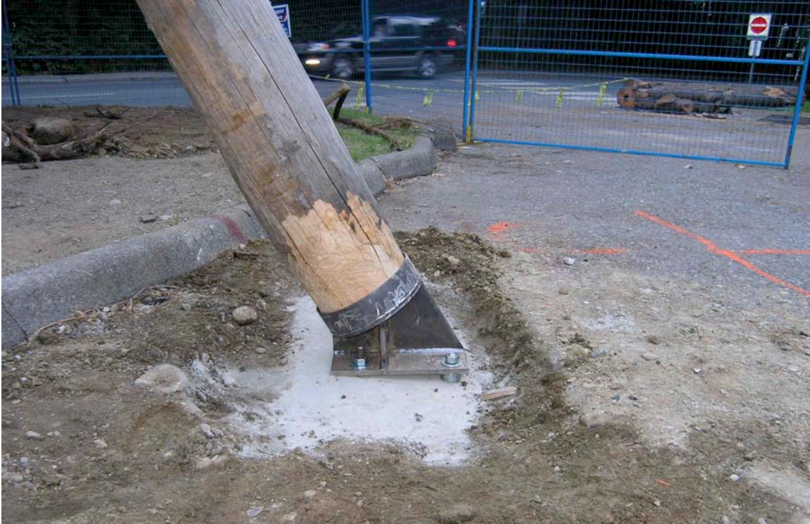
Figure 6. Base plate of north strut. (RAC July 25, 2008)
