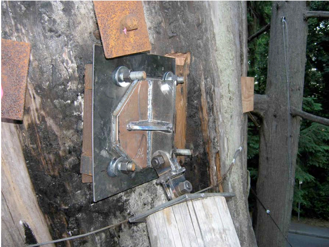
Figure 7. North strut top end universal bracket. (RAC July 25, 2008)
