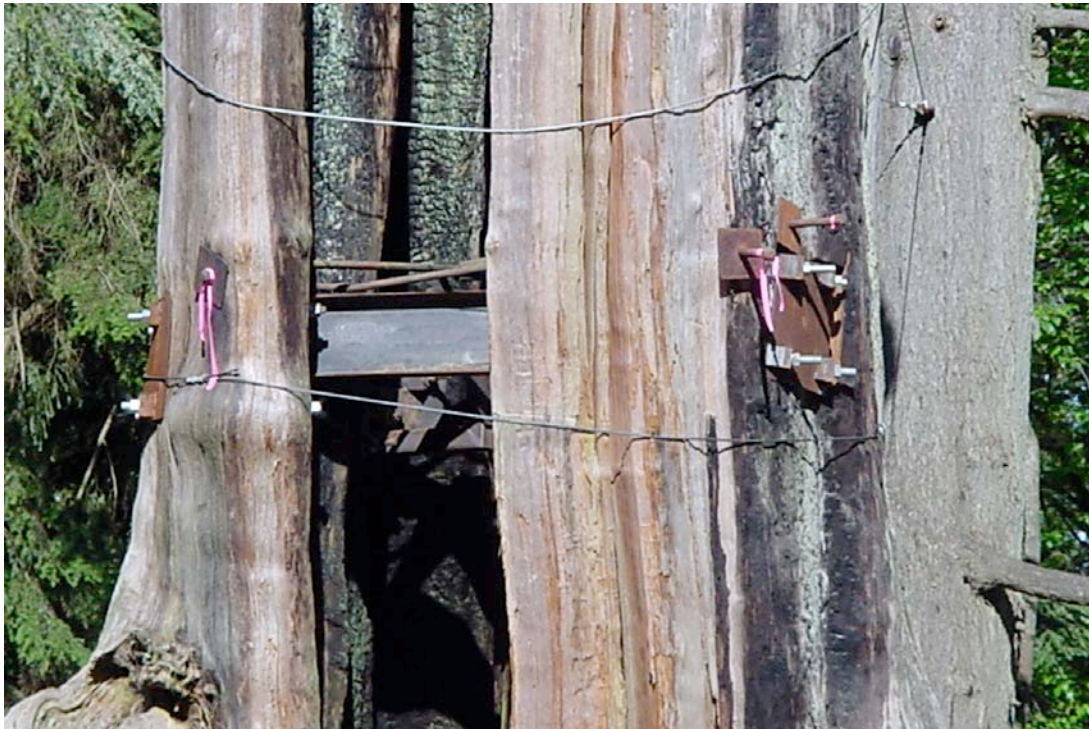
Figure 2. Mid-span steel internal support structure. (RC June 2008)
