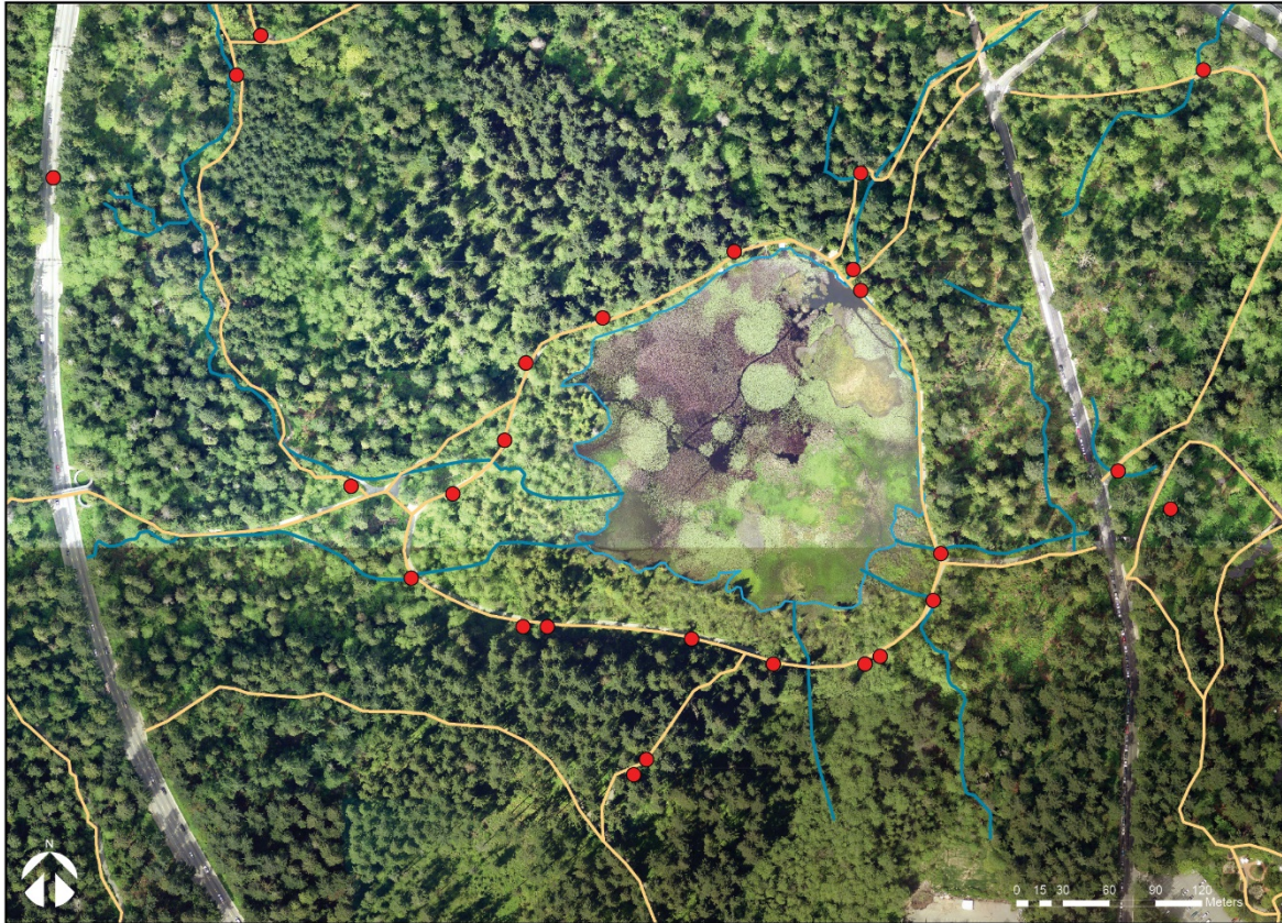
Figure 12: Illustration of existing culverts (red circles) in the vicinity of Beaver Lake.
