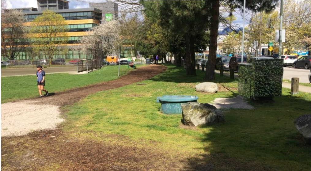
Figure 3 - Existing Glen Pump Station
