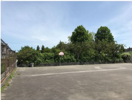
Existing sport court looking east
