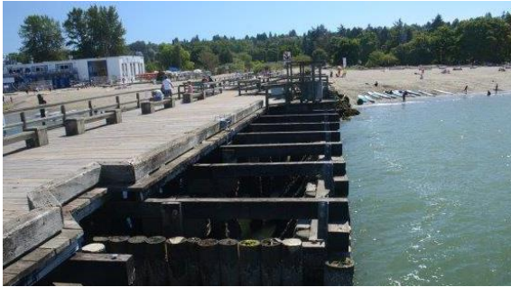
Aging pier structure
