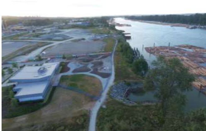
View east along Foreshore
