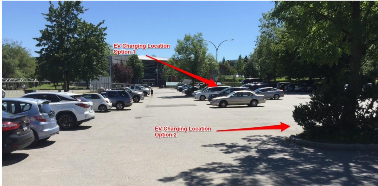
Figure 6: Photo of community centre parking area, facing south from anticipated BC Hydro connection point with the two possible location options for EV charging infrastructure noted in red.
