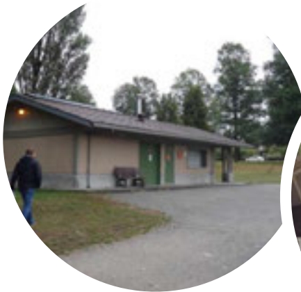
EXISTING: Trout Lake Little League washroom / concession building.
