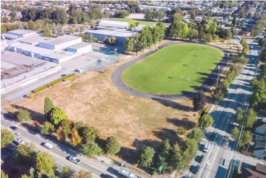
Figure 3: Existing Killarney Park Track and Field – Looking Northwest
