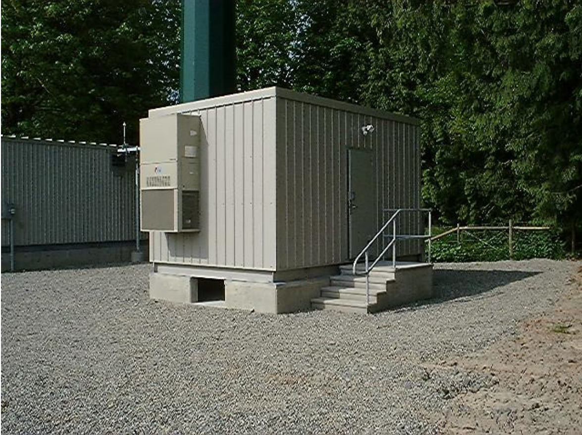
Rogers metal clad (11ft. x 17ft.) equipment shelter, door can be situated on the side as shown or the end of the building. The foundation can be set lower to be almost flush with grade.
