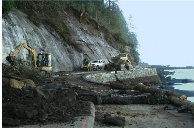
After debris was removed and basic repairs were done to the asphalt surface, public access to this portion of the seawall was re-established in November 2007. In the summer of 2008, major structural repairs were performed on the seawall between Prospect Point and Third Beach. The work was carried out while keeping the seawall open to the public.
