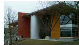
Millenium Sport Facility
