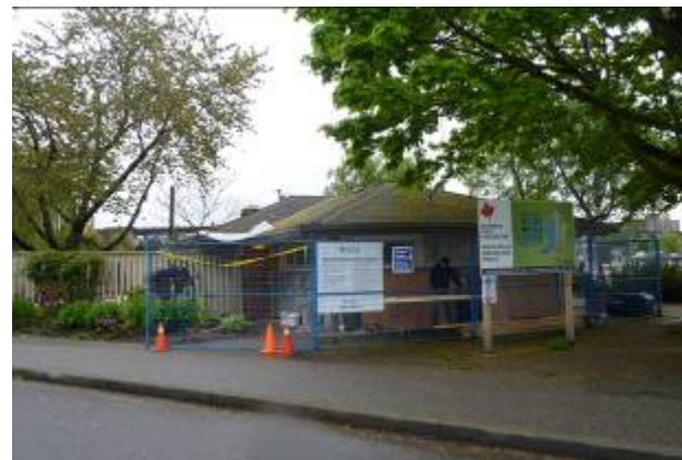
Washroom Renovations at Stanley Park Pavilion, Sunset Beach, Kitsilano Beach, Jericho Beach, and Chilco.
