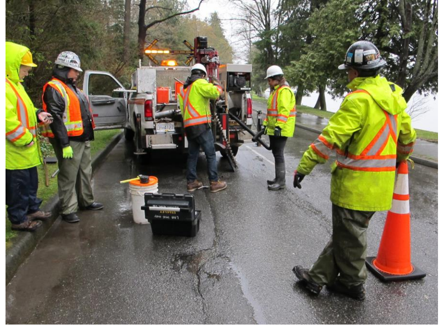
Stanley Park Drive – Pavement Testing Prior to Grinding/Paving
