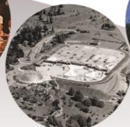
Concrete roof for reservoir 1965
