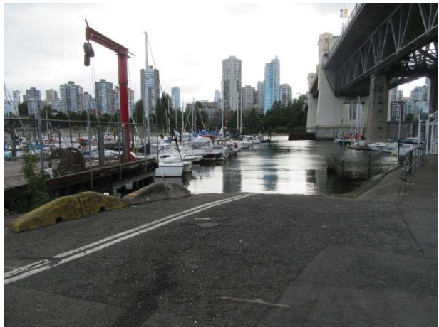
Burrard Marina crane area looking north
