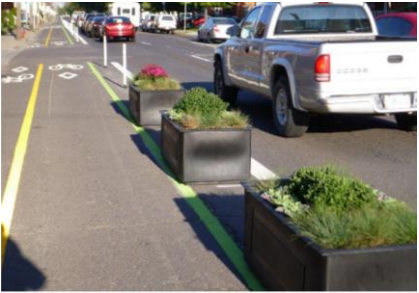
HAMILTON (Cannon Street pilot) Planters, pavement markings, signalization and signage, some bollards and rubber curbs, and street resurfacing.
