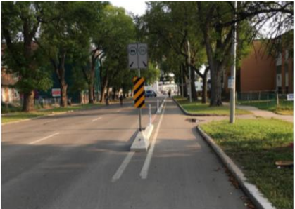
WINNEPEG (Sherbrook Street pilot) Pre-fabricated concrete barriers, bollards, pavement markings and signage. NOTE: Cost does not include installation.
