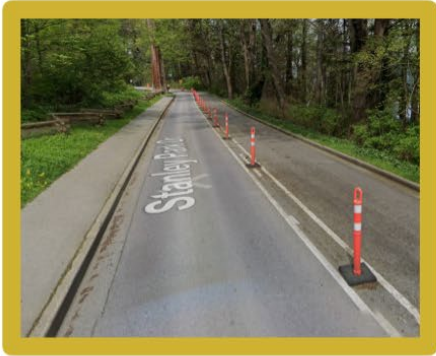
Delineators & Line Painting (double white line)
