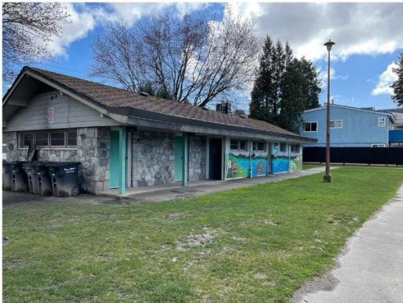
EXISTING FIELDHOUSE AND WASHROOMS
