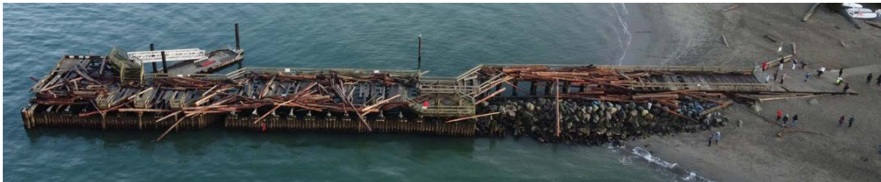
Fig. C: Log debris accumulated following January 2022 storm. Breakwater visible on near side of pier
