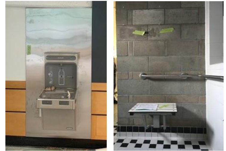
West End Community centre recently completed accessibility upgrades
