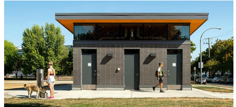
China Creek North Park Washrooms & Pump House
