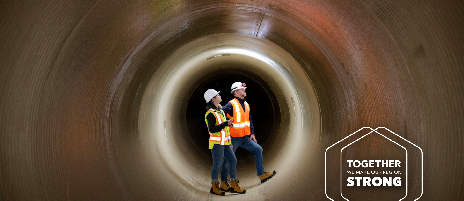
Second Narrows Water Supply Tunnel Construction
