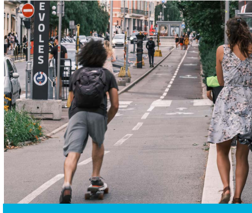
Raised crosswalk over a bike path in Nice, France helps improve compliance.
