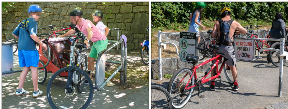
Figure 1: Example of Accessibility Challenges by Maze Gates on the Seawall
