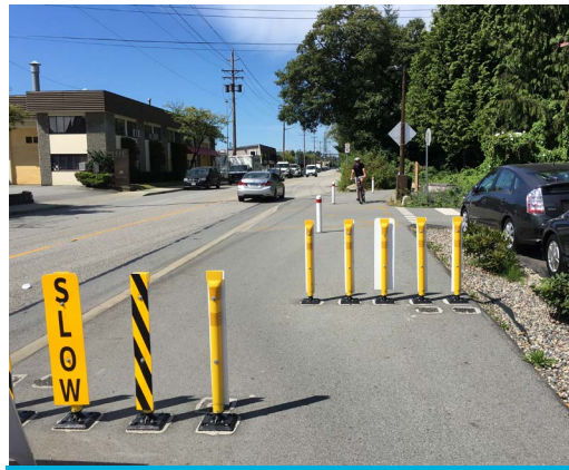
This chicane created using flexible posts achieves a similar effect to the maze gates but is spaced wider to allow for greater accessibility. It should be noted that this configuration is not well liked by cyclists.
