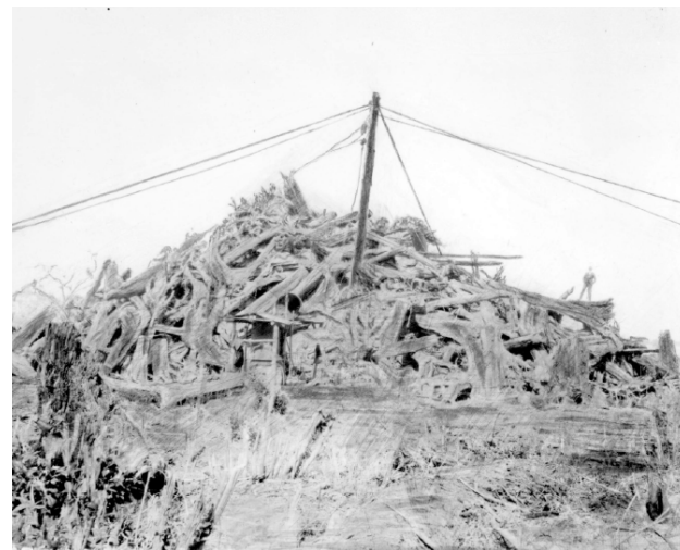
Figure 93. Clearing timber Quilchena 1926
