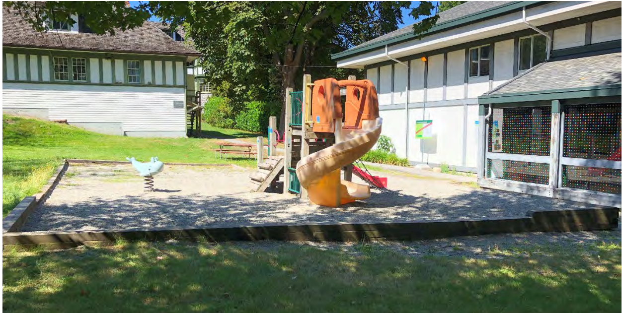
Previous playground condition looking northwest, summer 2022
