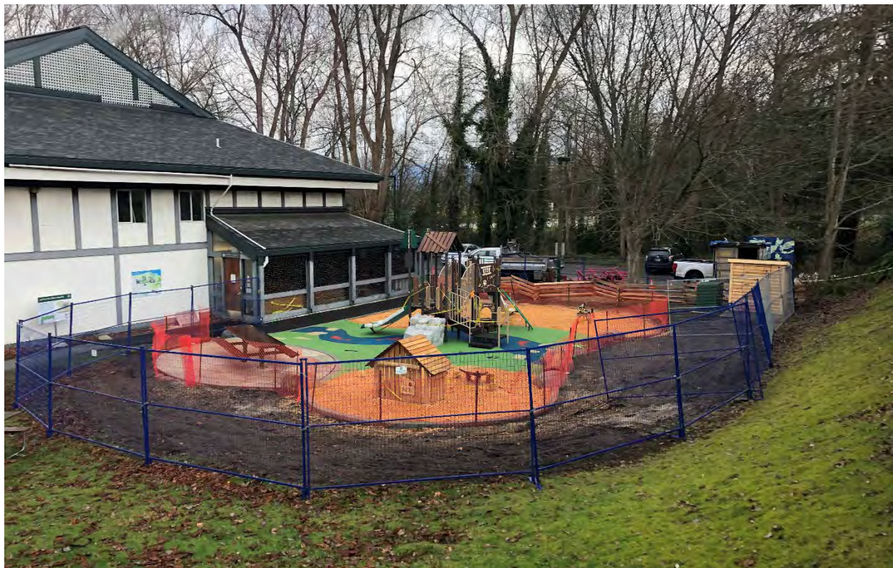
New playground under construction looking northeast, March 2023
