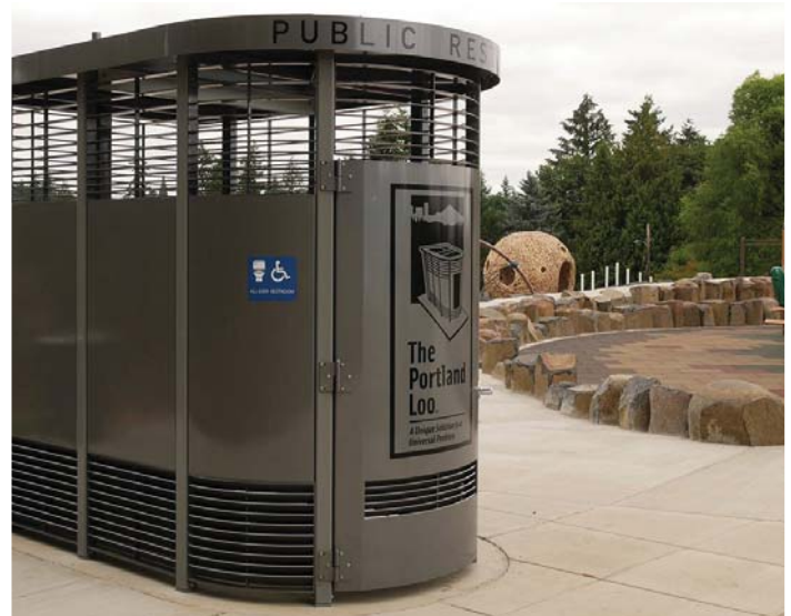
Portland Loo Installed
