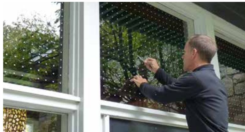
An example of a bird friendly retrofit in Vancouver.
