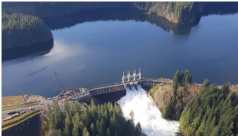
Figure 4 Hydro Generating Station at Campbell River [BC Hydro]
