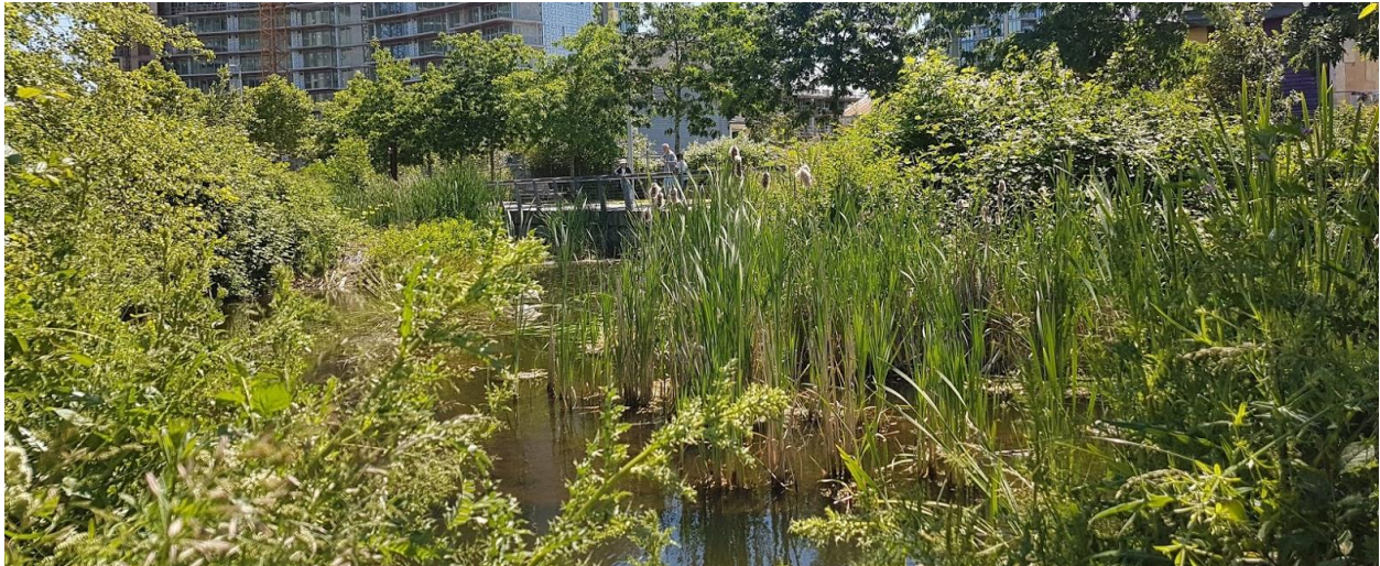
Figure 15: This wetland feature at Hinge Park helps to regulate stormwater flows and capture pollutants from runoff before draining into the Burrard inlet. (Photo taken by the author in Jun 2020).
